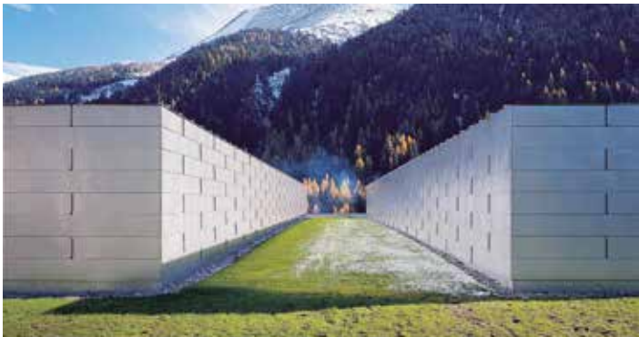
Roofinox Classic, Tartan flat-lock tiles special design, ARLBERG-well.com in St. Anton (1,284 m above sea level), Austria
